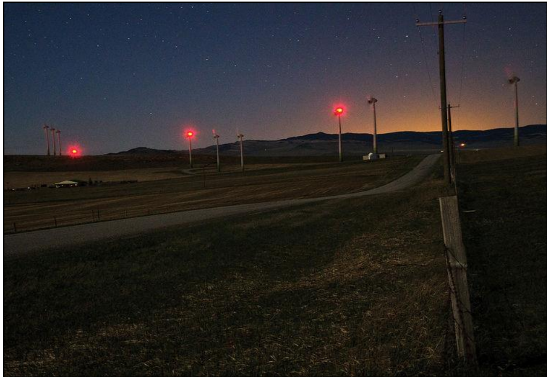
Figure 29: Aircraft warning lights fitted to the wind turbine hubs (Source: http://www.pinchercreekecho.com/2015/04/29/md-of-pincher-creek-takes-on-wind-turbine-lights. )
