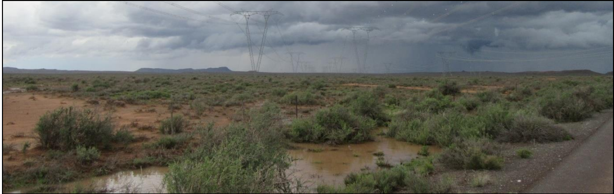
Photograph 3.4: Four (2 X 400 kV and 2 X 765 kV) Tx lines traversing the Hutchinson Road within a 350 m corridor on Annexe Rondawel
