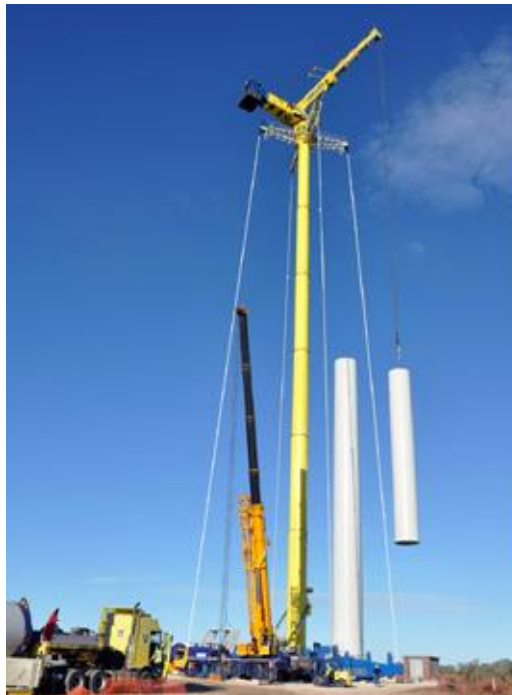
Figure 2-6: Example - Cranes at work
