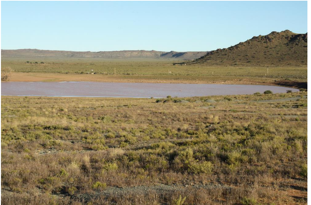
Figure 3: An example of a large dam at the project site
