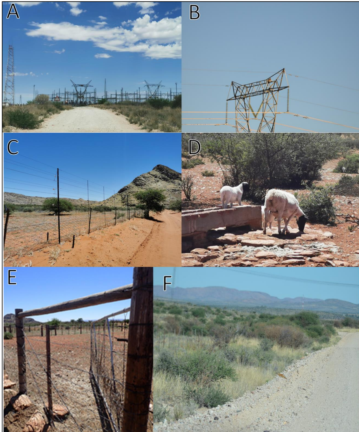
Figure 8-1 Some of the identified impacts within the project site; A) Existing substation with associated powerlines, B) High voltage powerlines, C & E) Fencing, D) Livestock and E) Roads and Cell phone towers
