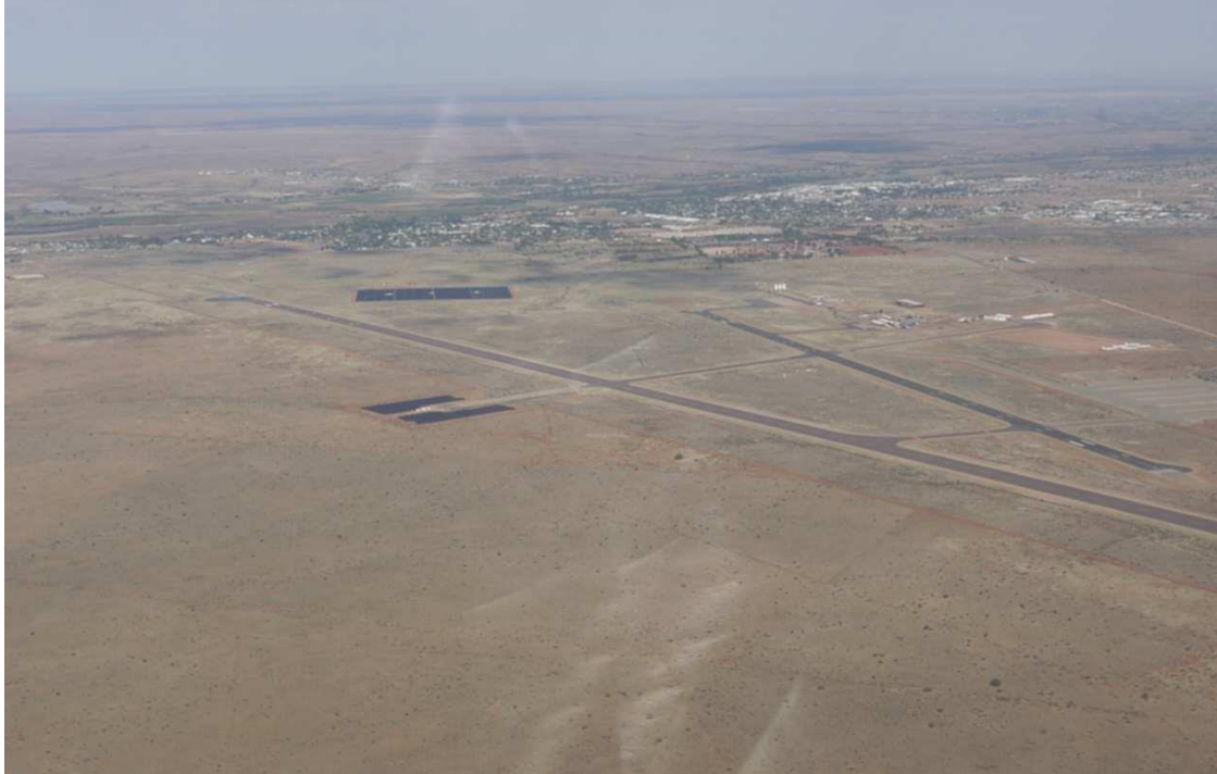
PLATE 14, EXISTING SOLAR ARRAYS AT UPINGTON AIRPORT AS SEEN FROM THE AIR
