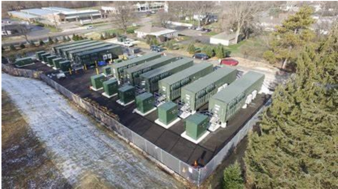
PLATE 3 - TYPICAL BATTERY ENERGY STORAGE SYSTEM
