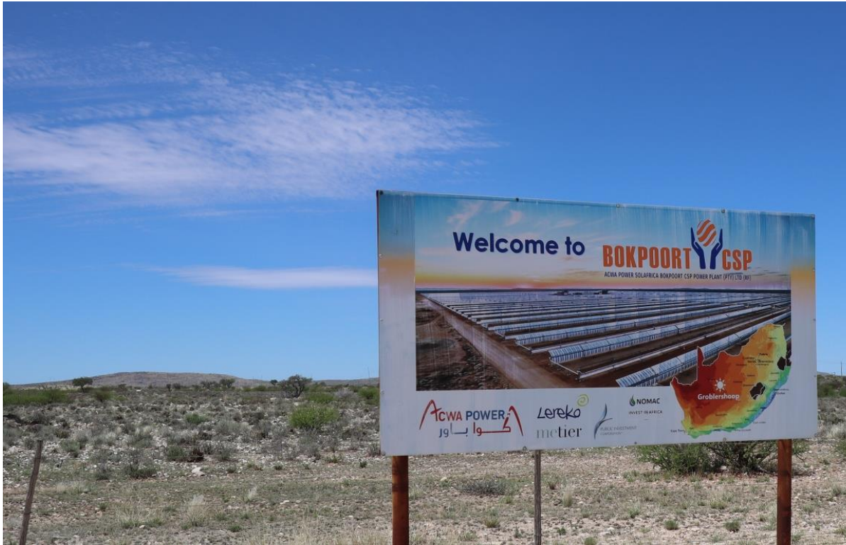
PLATE 4, THE BOKPOORT CSP SOLAR PROJECT
