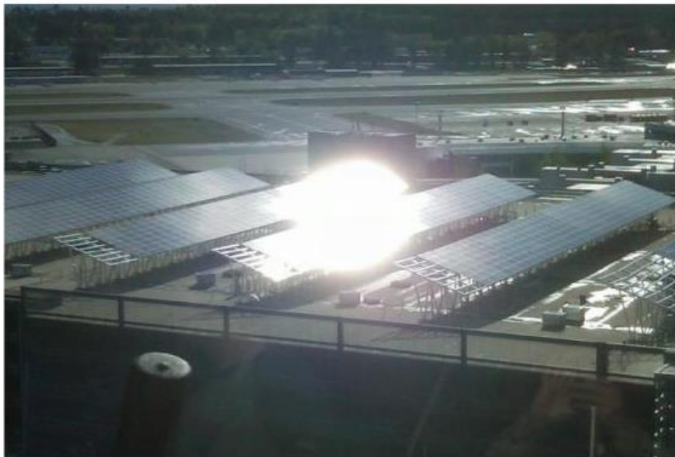
PLATE 18 - GLARE EXPERIENCED IN THE CONTROL TOWER AT BOSTON REGIONAL AIRPORT FROM A PV ARRAY
