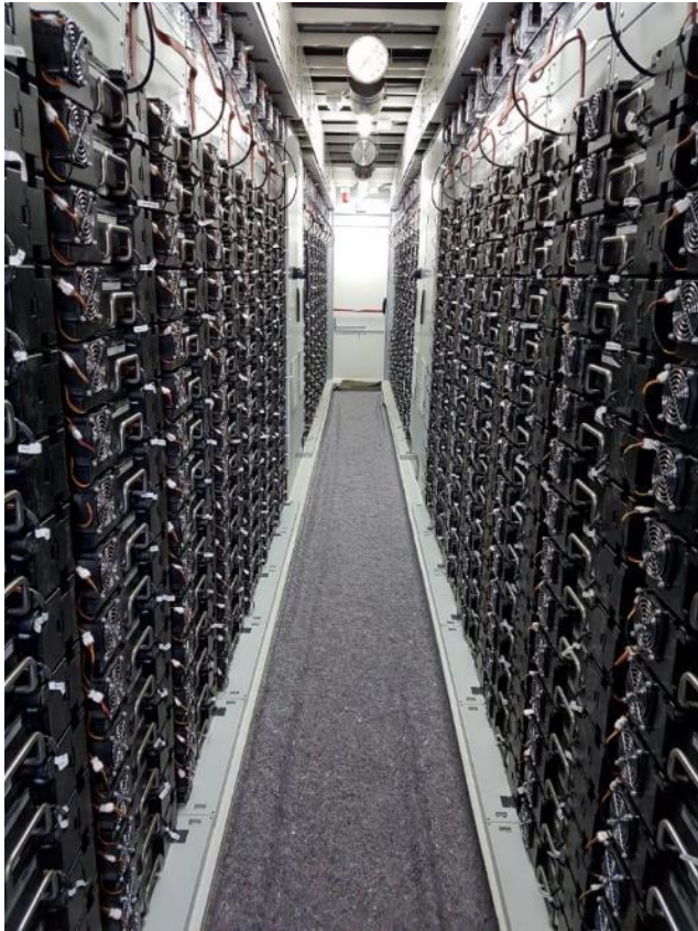
Figure 2.10: Li-Ion BESS internal design and implementation of a container used within a BESS. The image shows a series of sealed battery cell packs within a containerised module (Source: Enel Green Power).
