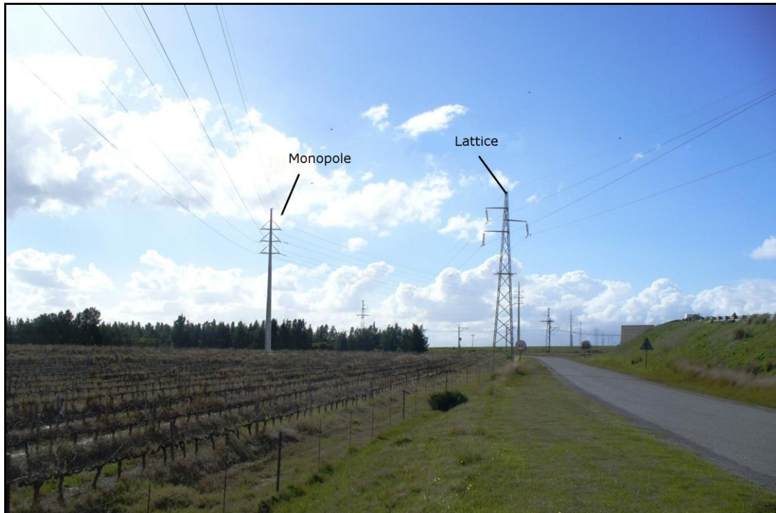
Figure 3: Longer distance view of power line towers.
