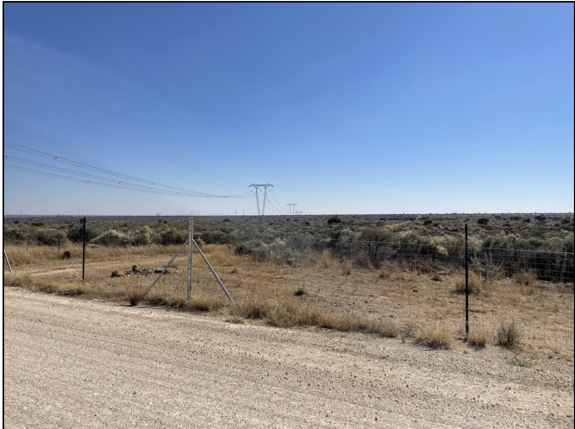
Figure 12: The Mercury to Mookodi 1 400kV power lines near the Waterloo Solar PV facility.
