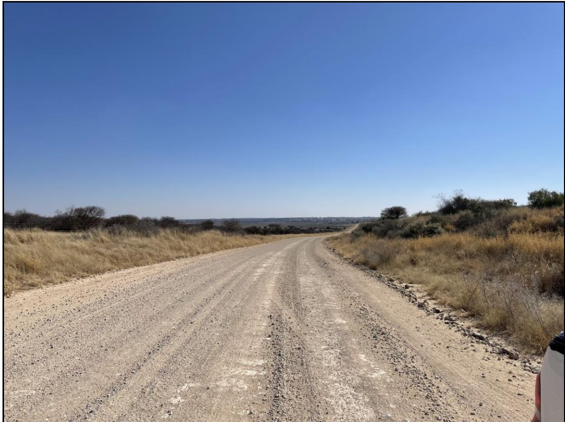
Figure 10: View from the northern ridge looking back towards Vryburg. (Note: The power line will traverse west (left) of this road).
