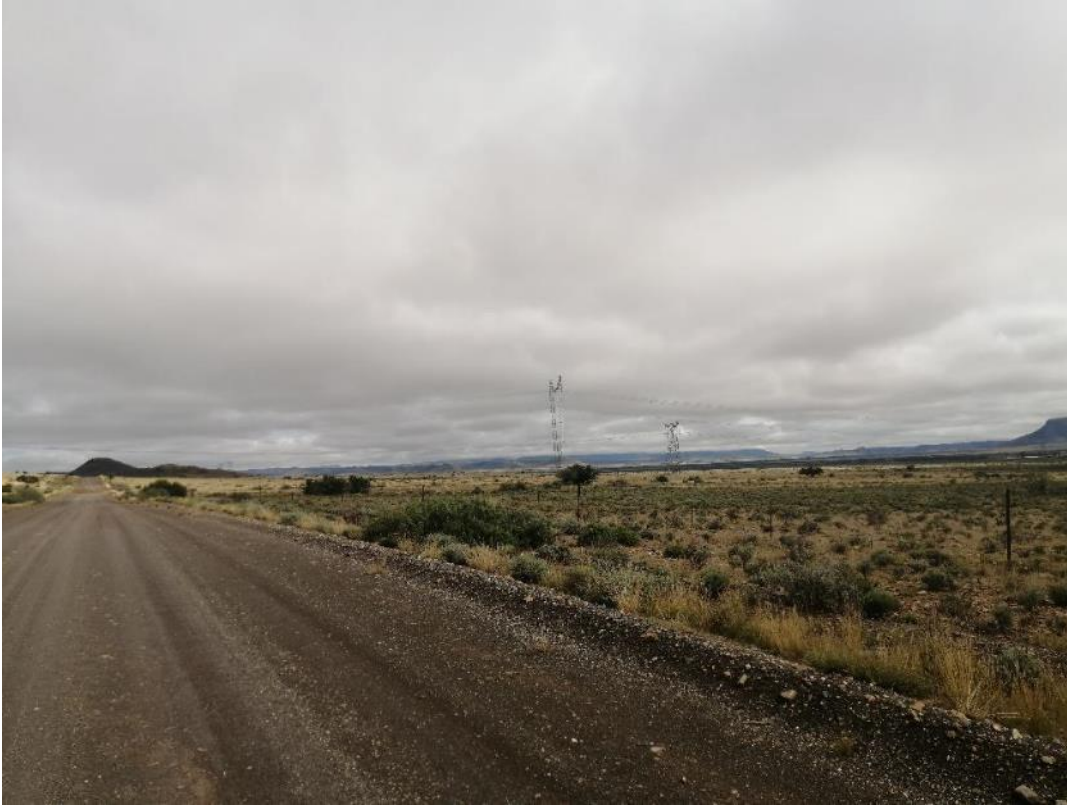
Figure 9: Droerivier/Hydra powerlines to the west of the site
