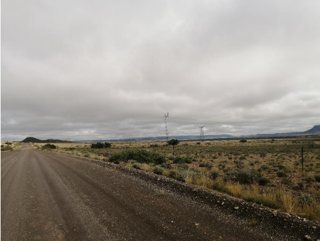
Figure 8: Droerivier/Hydra powerlines to the west of the site
