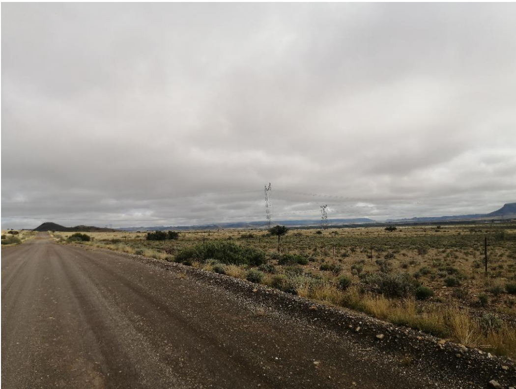
Figure 8: where the OHL will cross the existing Droerivier/Hyra 1&3 400 kV OHL before connecting to substation B
