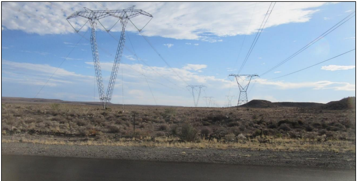
Photograph 3.6: Existing 2 x 400 kV line corridor traversing the R61 approximately 5.6 km south-east of Beaufort West
