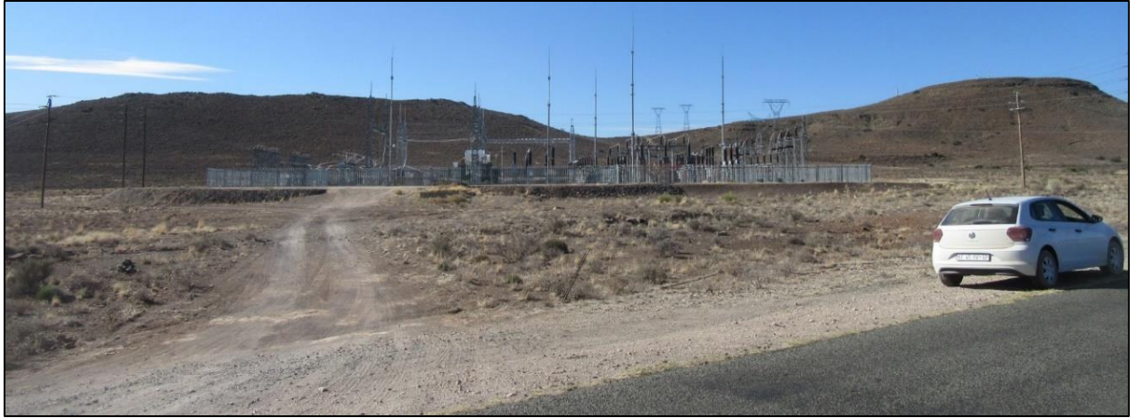
Photograph 3.5: Eskom substation located along the Hopewell Road
