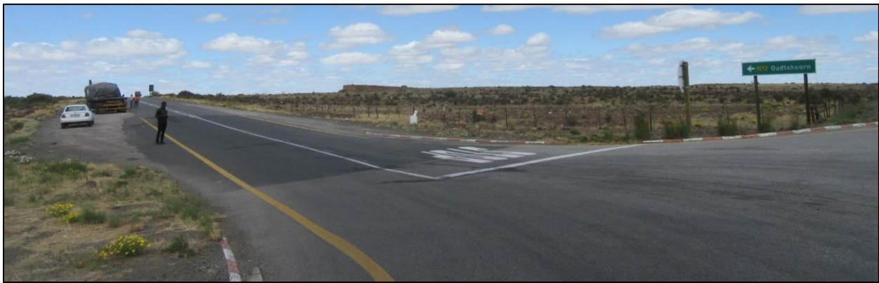
Photograph 3.1: Intersection of the N12 with the N1 ~3 km north of Eskom's Droeërivier MTS
