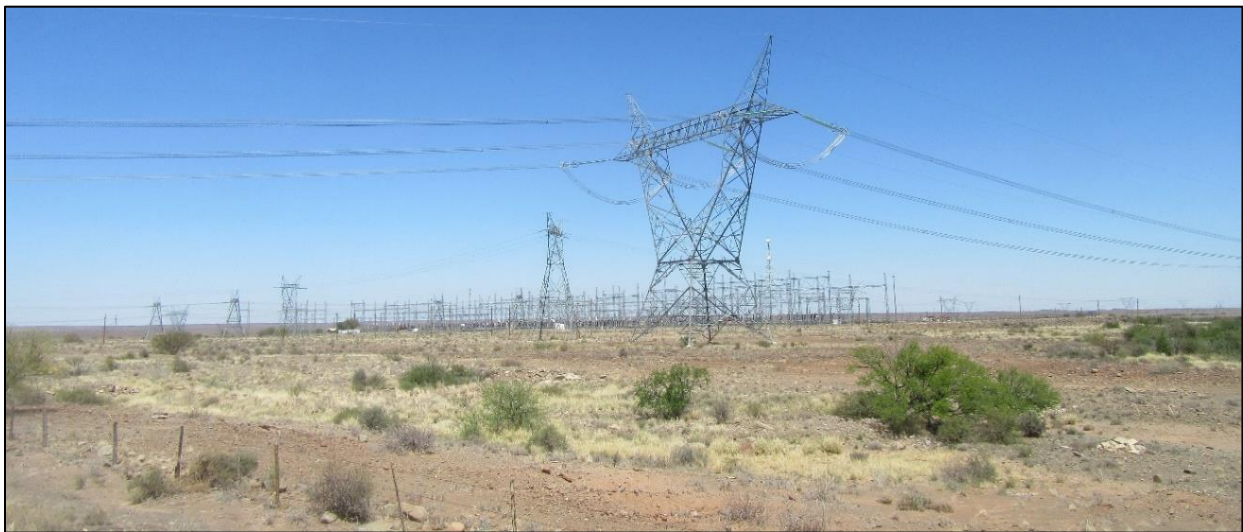
Photograph 3.4: Eskom's Droeërvier MTS, seen from the north from along the N12
