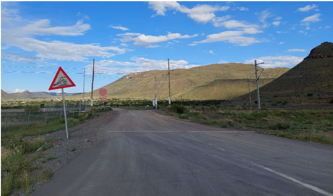
Photo 3-1: Intersection on MR587 at level crossing
