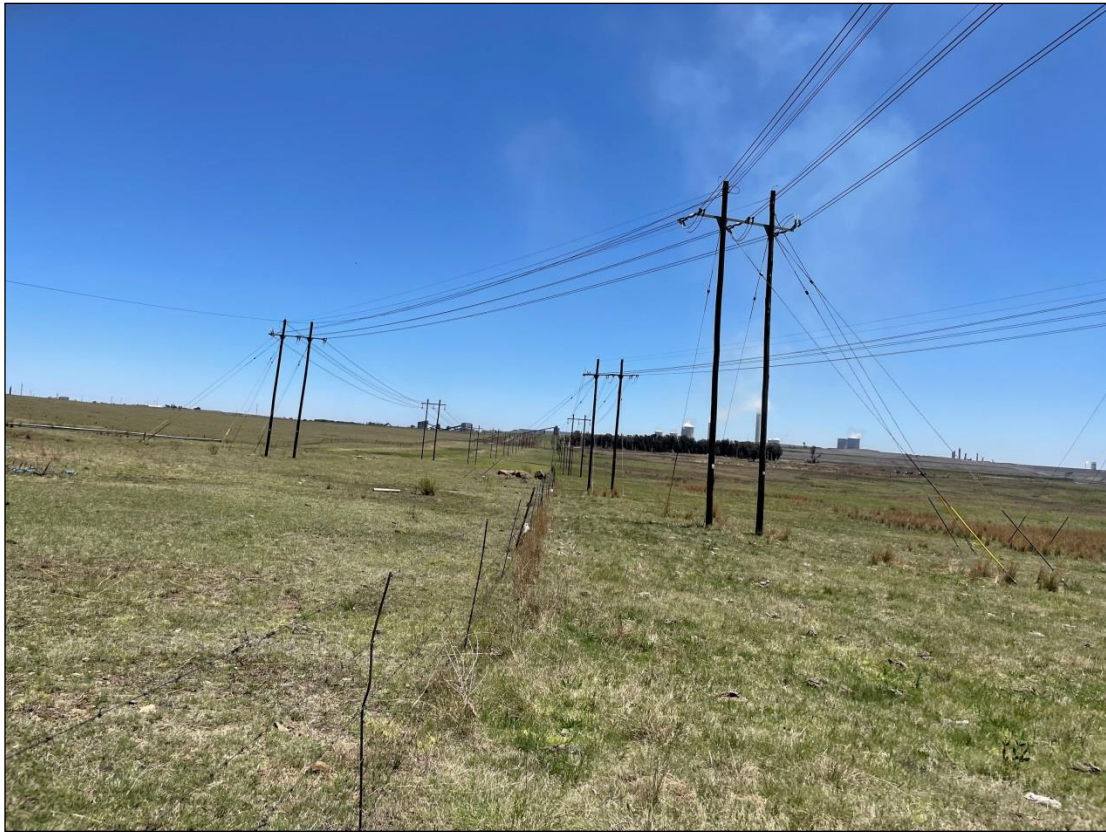
Figure 7: Existing power lines near the site.
