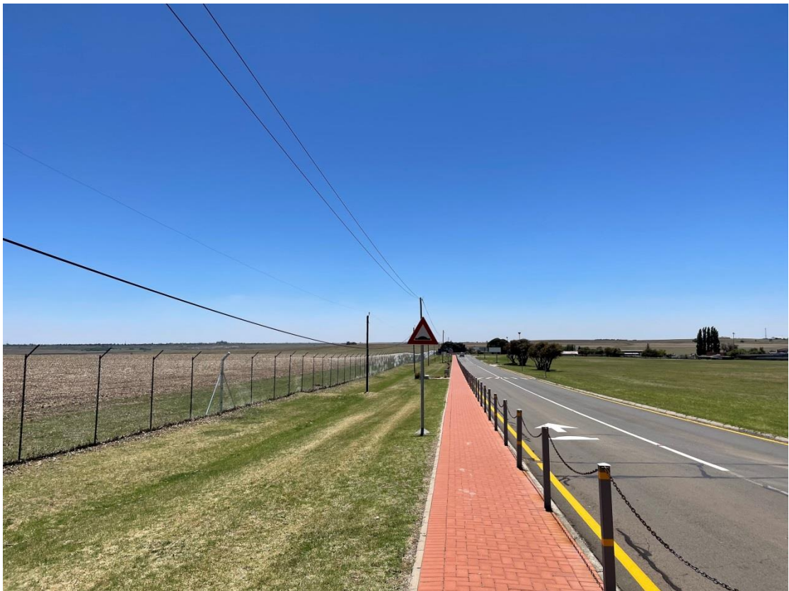
Figure 10: Access road to the Riaan Rademan Training Facility. (Note: the PV arrays will be immediately adjacent to the fence).
