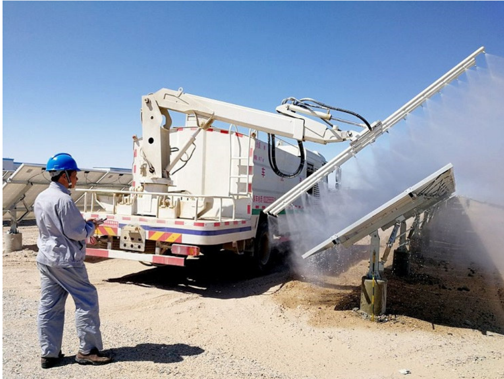
Figure 7-1: Mechanical Solar panel cleaning system
