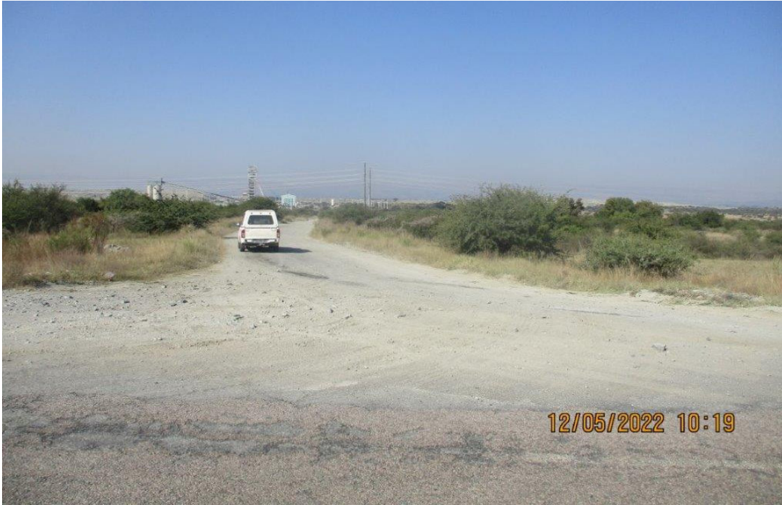
Figure 5-7: Private Road north approach
