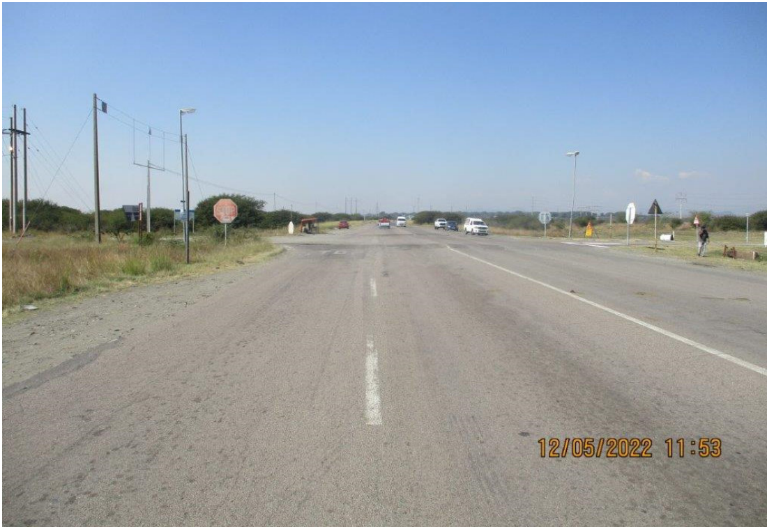
Figure 5-5: D108 northwest approach
