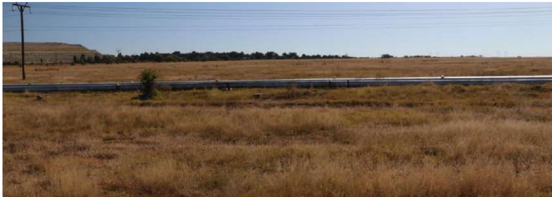
Figure 16: Surface infrastructure such as pipelines, dirt roads and ditches all act as obstruction to surface flow and will also contribute toward the modification of surface runoff patterns.
