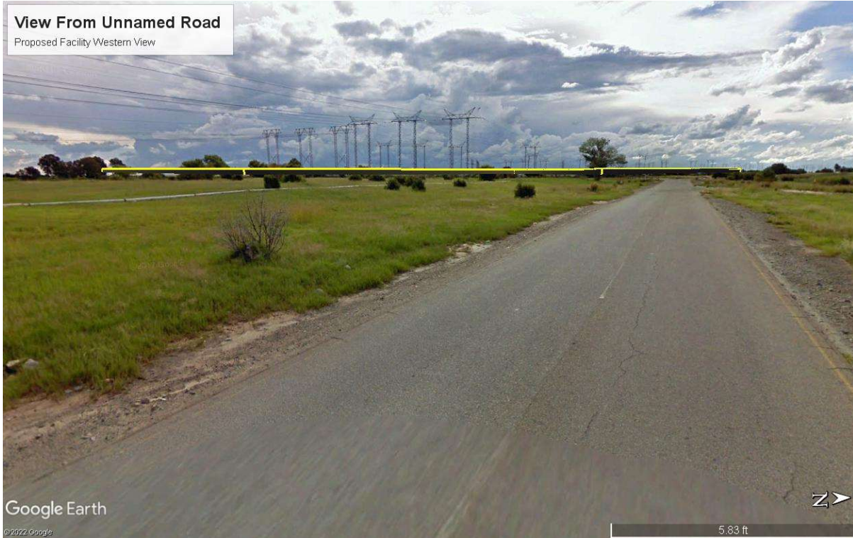
Figure 4: Western View of PV facility
