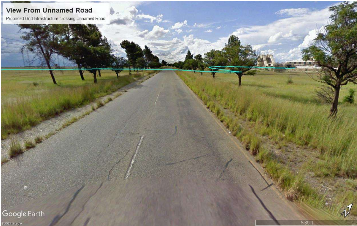
Figure 6: Gridline Road Crossing
