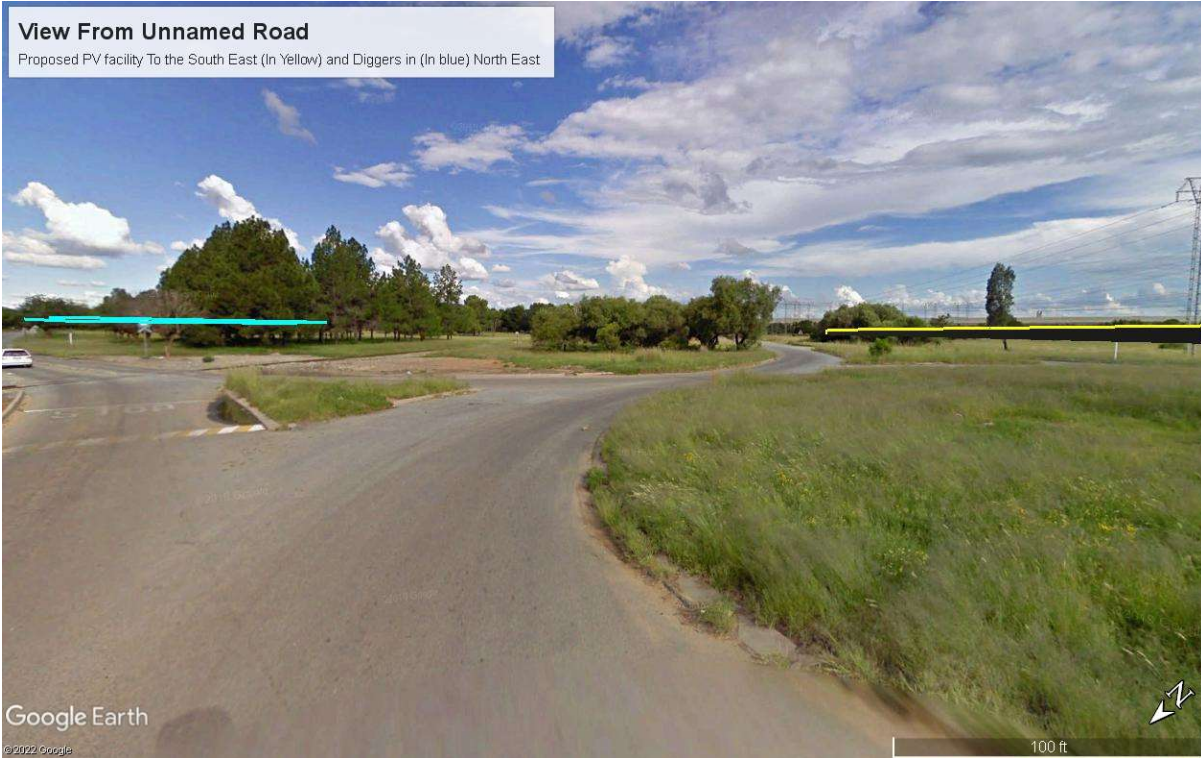
Figure 8: View of Diggers in and PV facility
