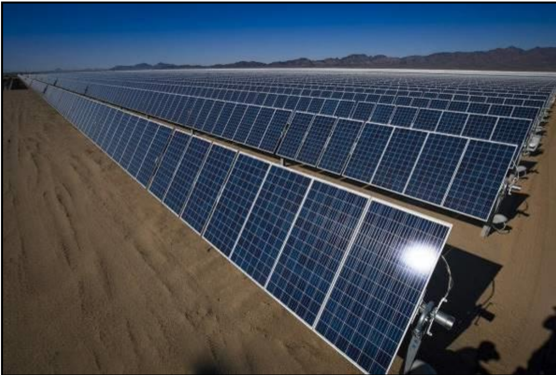
Photograph 1.1: Typical PV SEF facility
