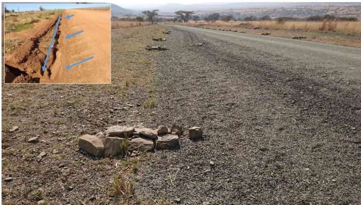
Figure 6-3 Example of road margin erosion prevention
