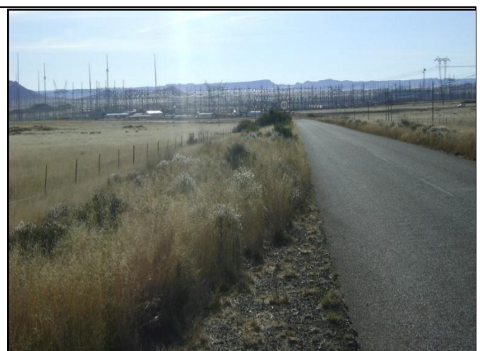
The Hydra Substation in the west of the study area.
