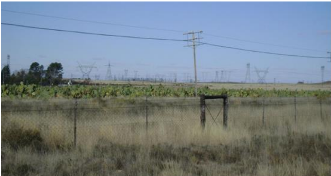
Figure 9: Power line infrastructure along the N10 national road.
