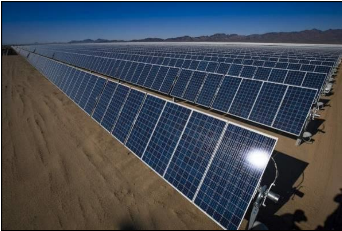
Photograph 1.1: Typical PV SEF facility
