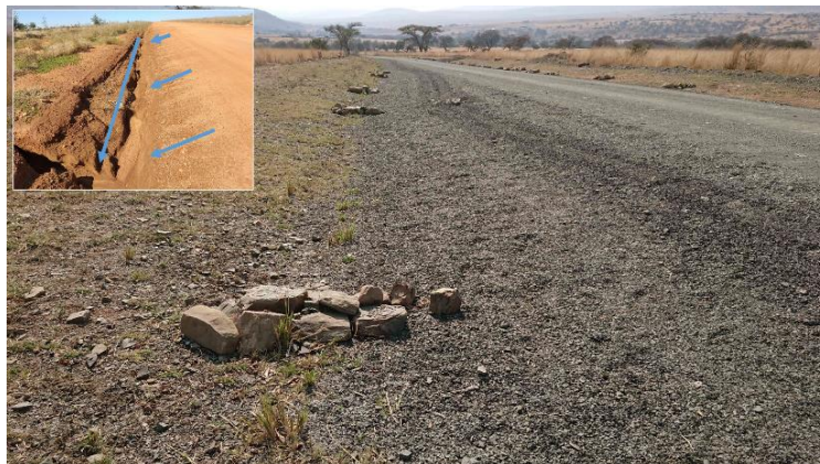
Figure 6-3 Example of road margin erosion prevention
