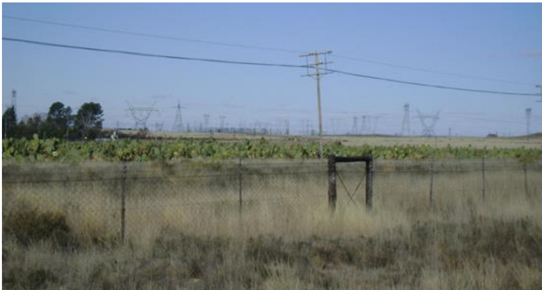
Figure 9: Power line infrastructure along the N10 national road.
