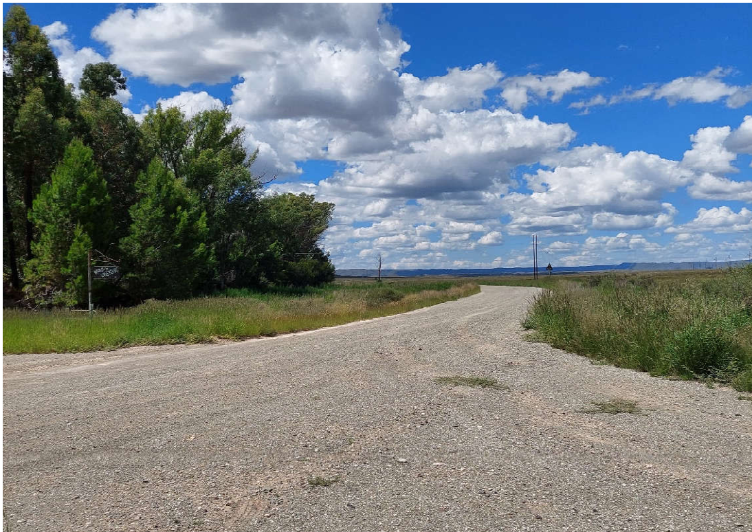
Photo 3-3: Insufficient shoulder sight distance to the East on proposed access to Riet Fountain Solar PV1
