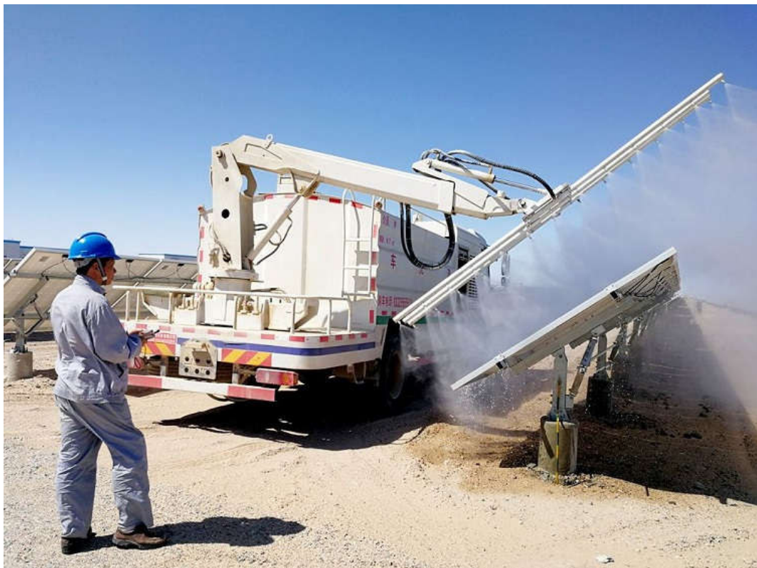
Figure 6-1: Mechanical Solar panel cleaning system
