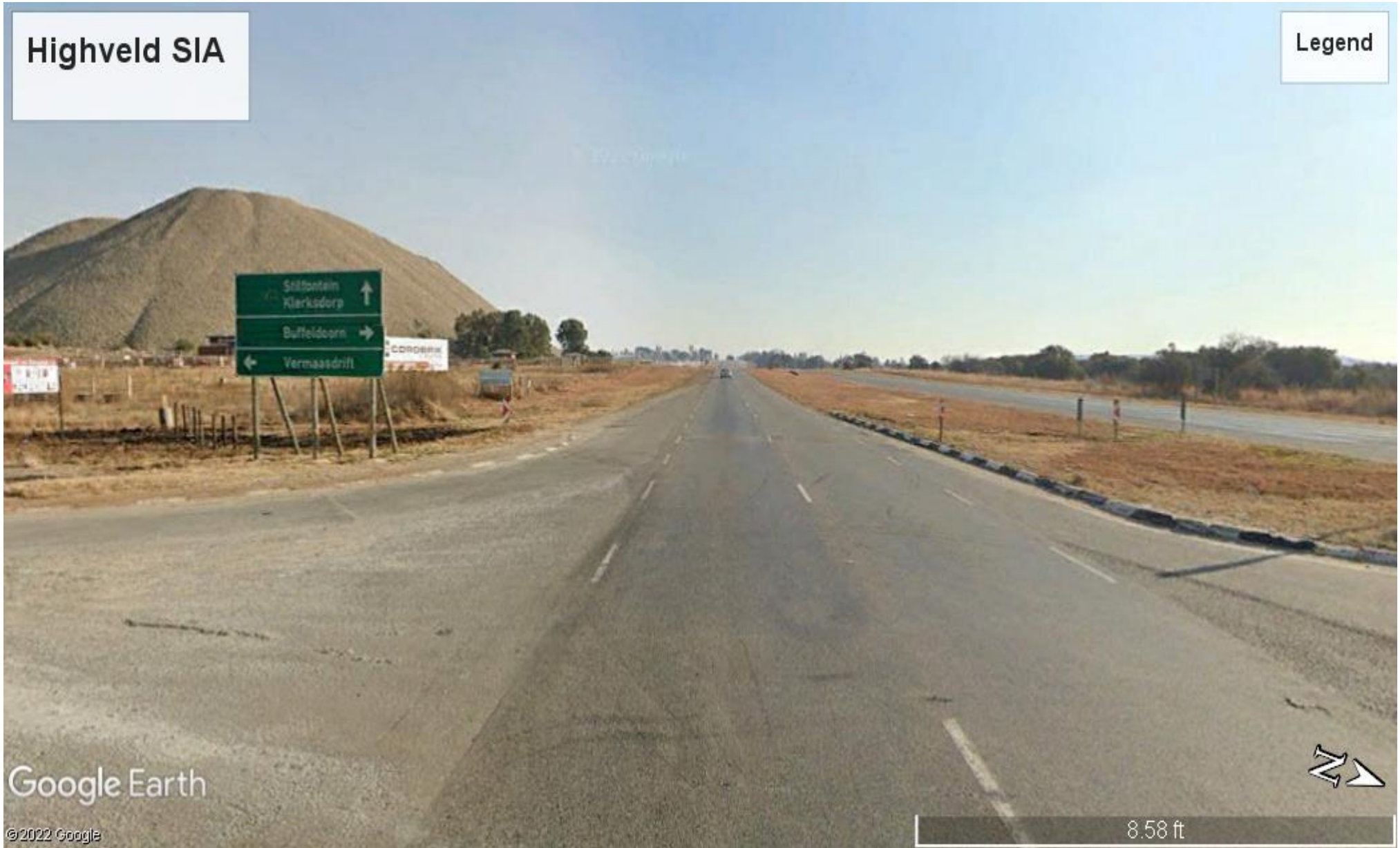
Figure 1.3. Ground view of N12 into access road
