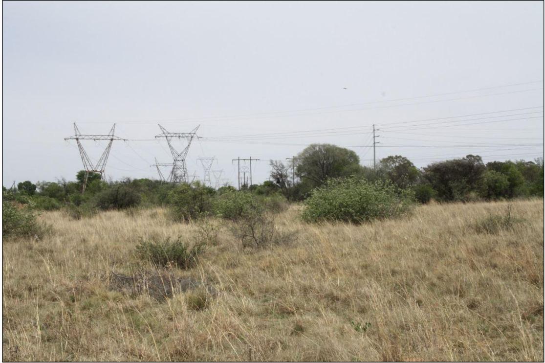
Figure 8: Power lines near the Watershed Substation.
