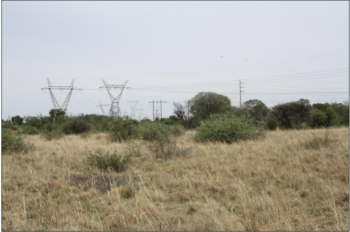
Figure 8: Power lines near the Watershed Substation.
