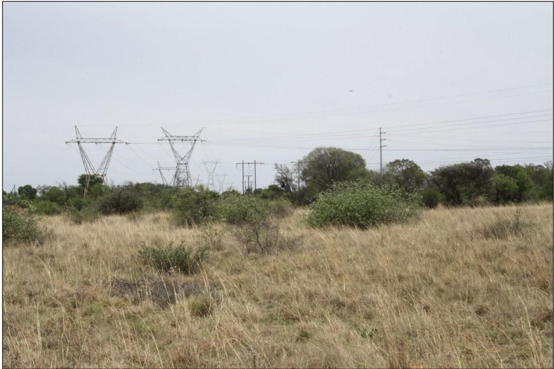
Figure 8: Power lines near the Watershed Substation.
