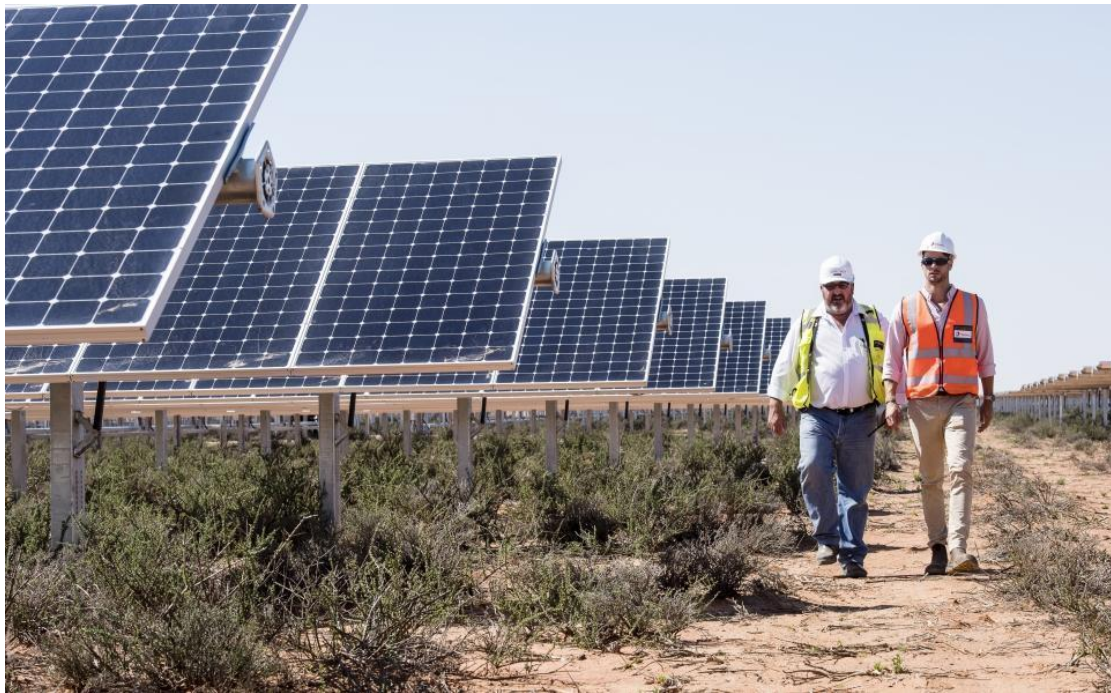
Figure 2: Photovoltaic (PV) solar panels. (Photo: SunPower Solar Power Plant – Prieska).
