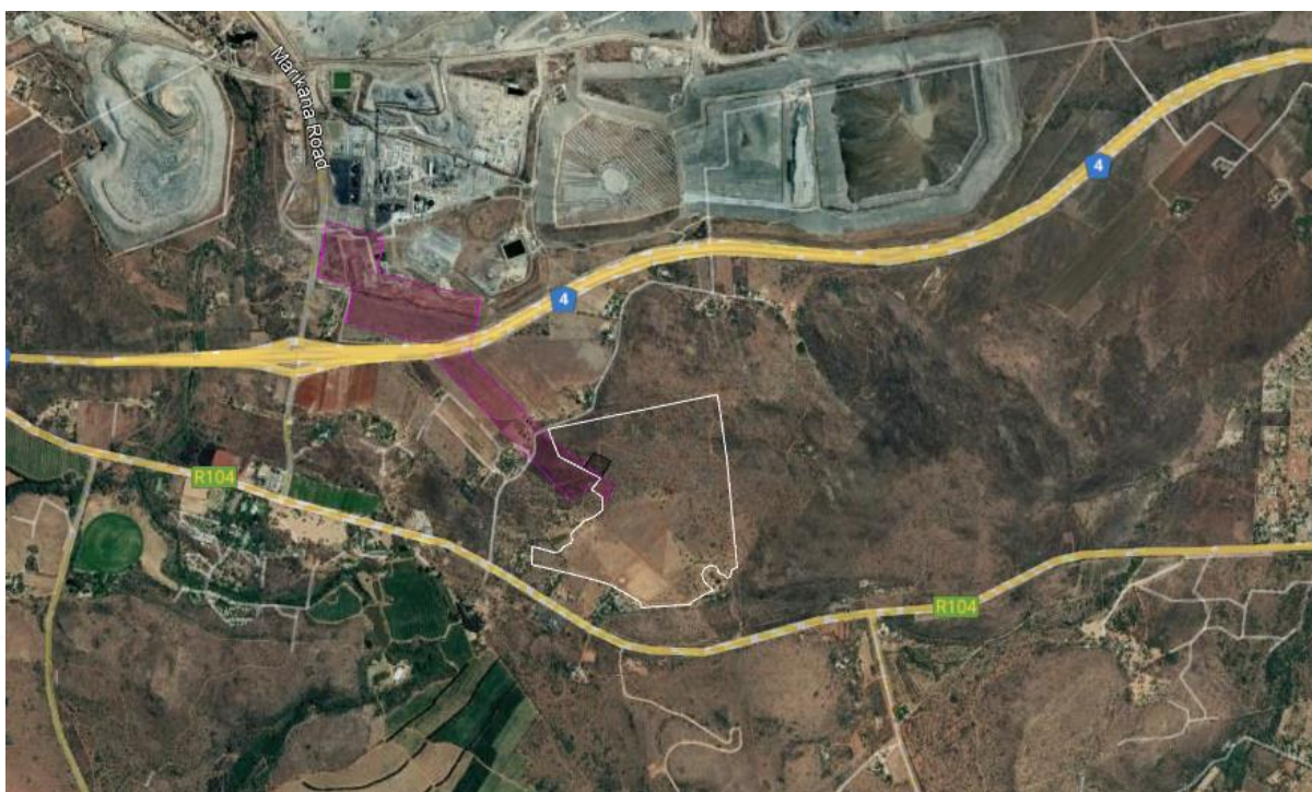
Figure 2.1: Location of the R104, N4 and Marikana Road in relation to the Project.
