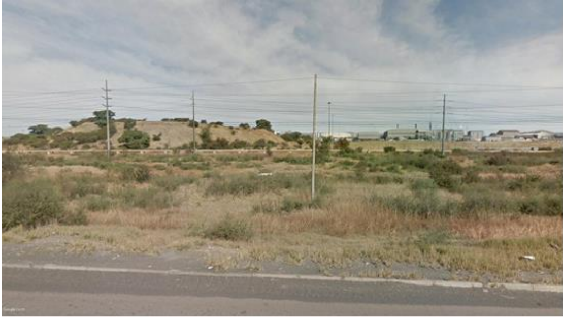
Figure 11: Mine dumps, power lines and mining infrastructure within the Study Area.
