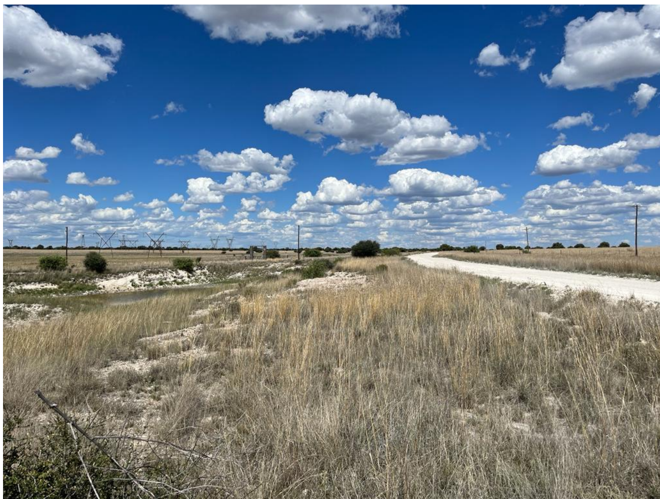
Figure 6: Various powerline infrastructure
