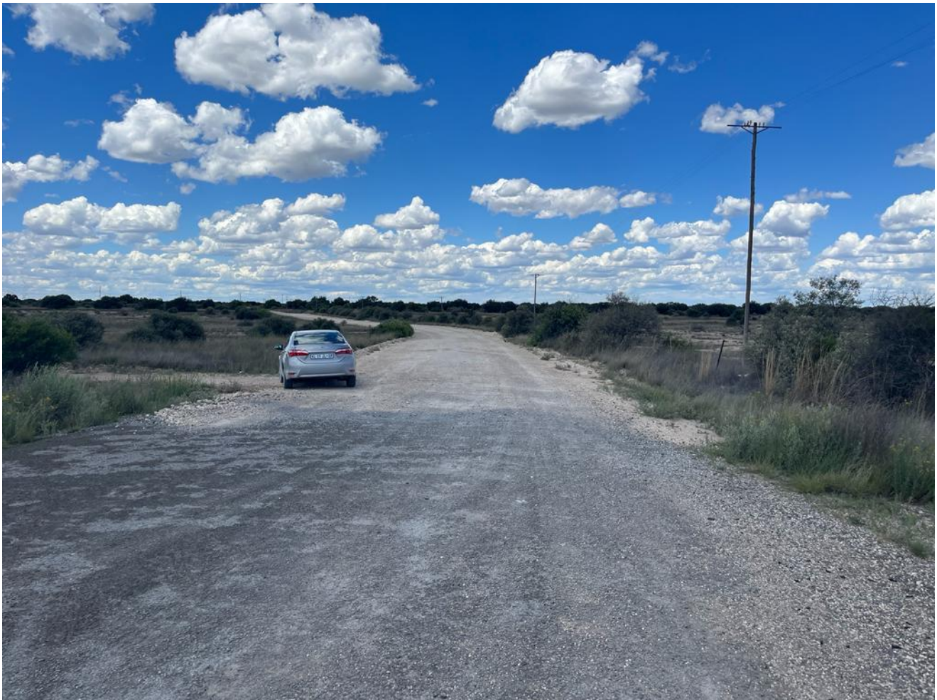
Figure 5: Access to the site via the secondary road
