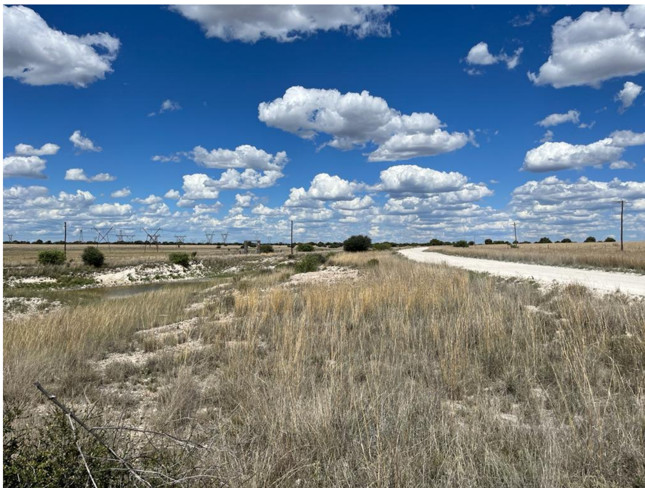
Figure 6: Various powerline infrastructure
