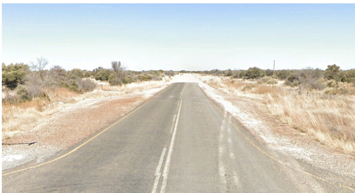
Figure 4-16: Views on R385 in southern direction at intersection with gravel road
