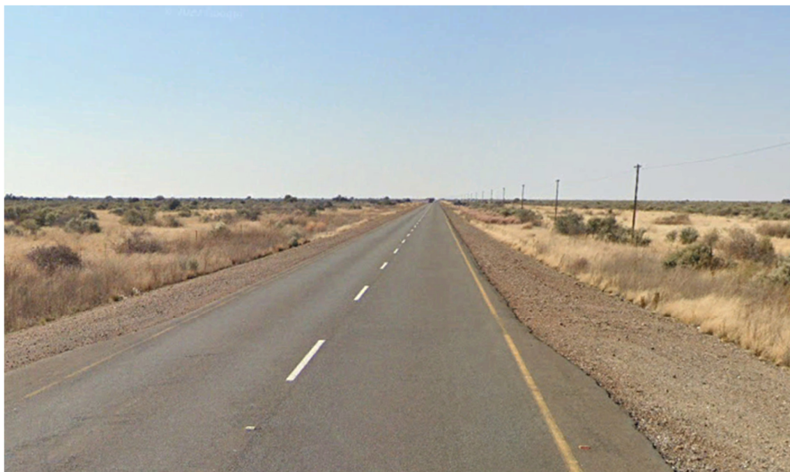
Figure 4-8: View in eastern direction on R31 at intersection with gravel road
