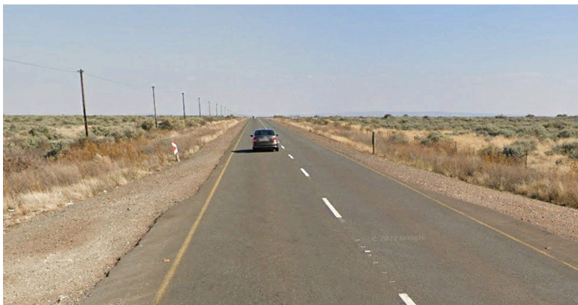
Figure 4-7: View in western direction on R31 from intersection with gravel road
