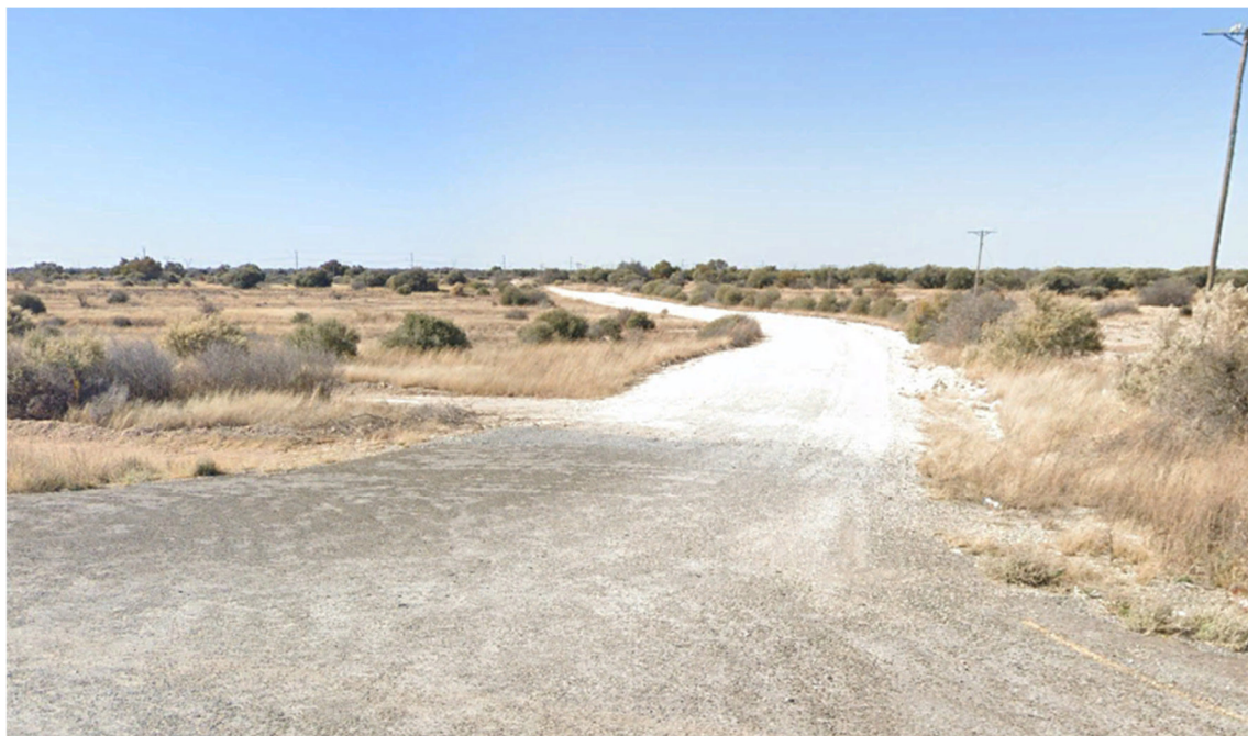
Figure 4-15: Intersection of R385 and gravel road towards site
