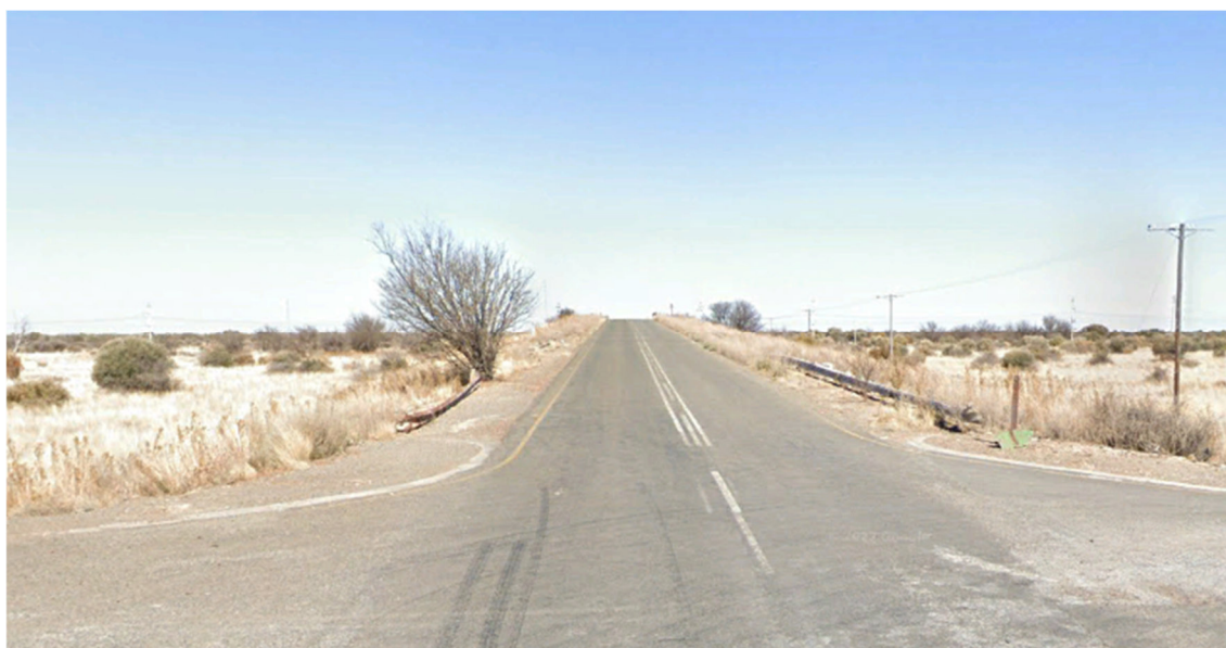
Figure 4-12: View on R385 in a southern direction from the intersection with the gravel road
