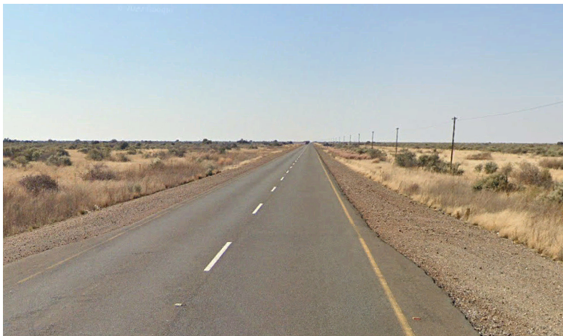
Figure 4-8: View in eastern direction on R31 at intersection with gravel
