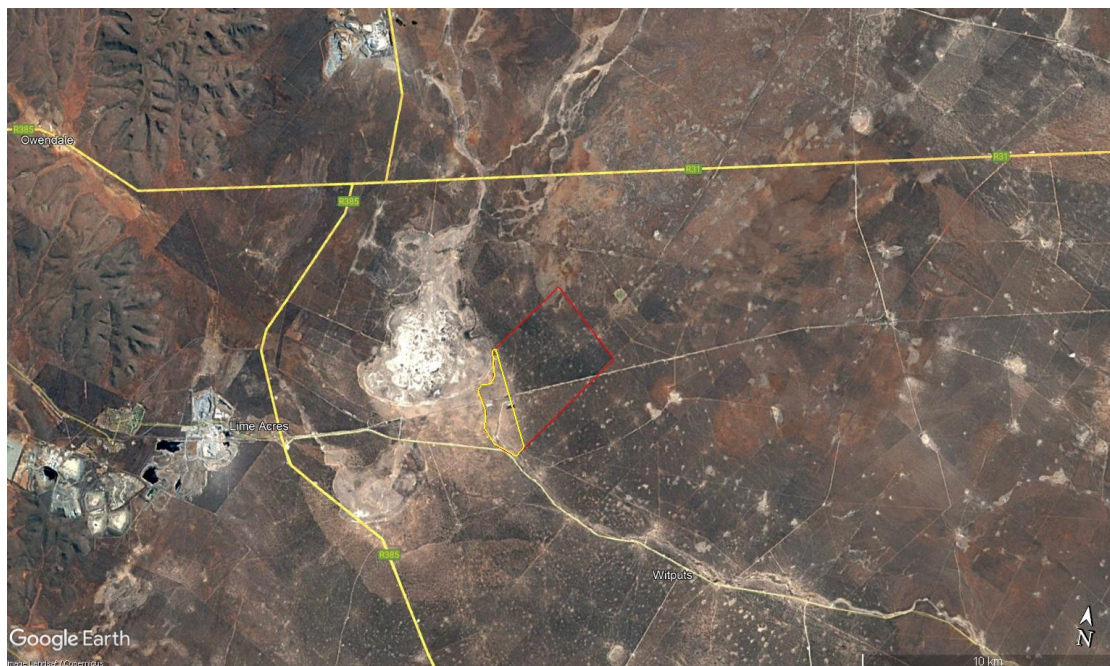
Figure 5: Limestone PV1 Solar Facility property.
