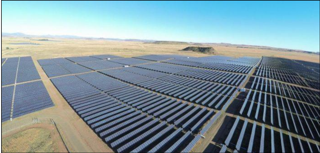
Figure 2: Aerial view of PV arrays. (Photo: Scatec Solar South Africa).
