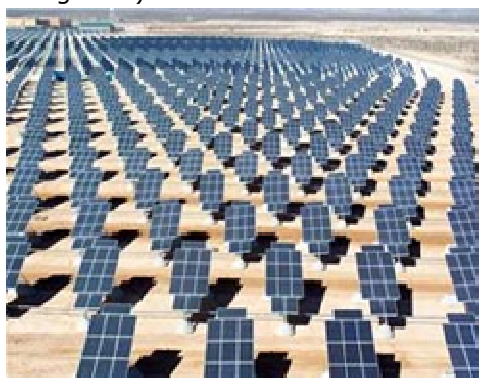
Figure 3: Figures showing a typical PV cell and an array of PV panels, where each panel is generally up to 3 m high.
