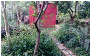
SIDE VIEW OF EX. OUTBUILDING
