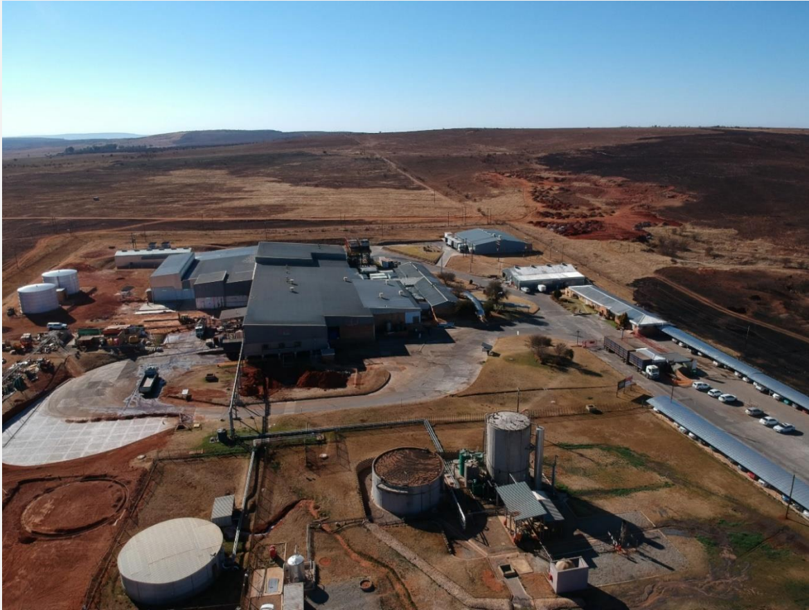
Figure 1: Processing Plant prior to the expansion of the live bird receiving area, air-line chiller and gyro freezer
