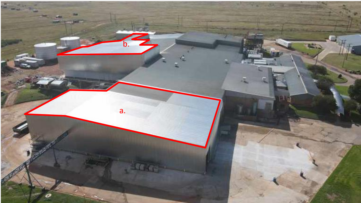
Figure 2: © Provided by Saturday Star - 24 Jun 2022 - (a.) Processing Plant post expansion of the (a) live bird receiving area and (b), Air-line Chiller and Gyro Freezer
