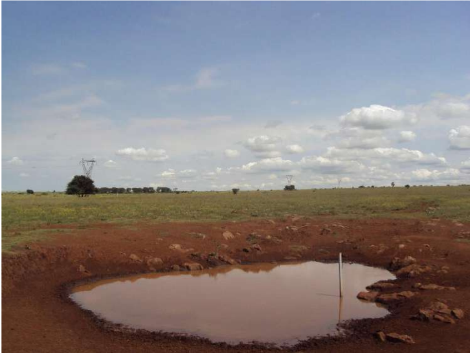
Figure 4: View showing excavation for livestock waterhole on the west section of the project footprint
