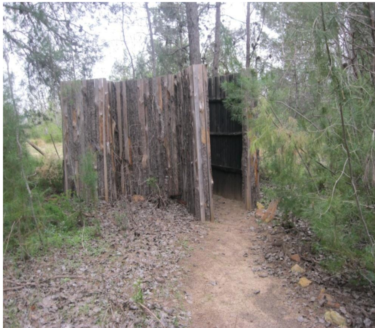
2.10: Existing toilets at the camp sites.
