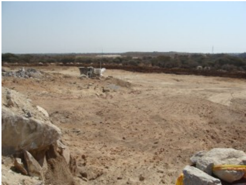
Figure 5: Another view of the site.
