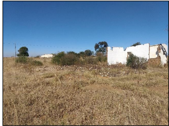
Remains of Mine House
