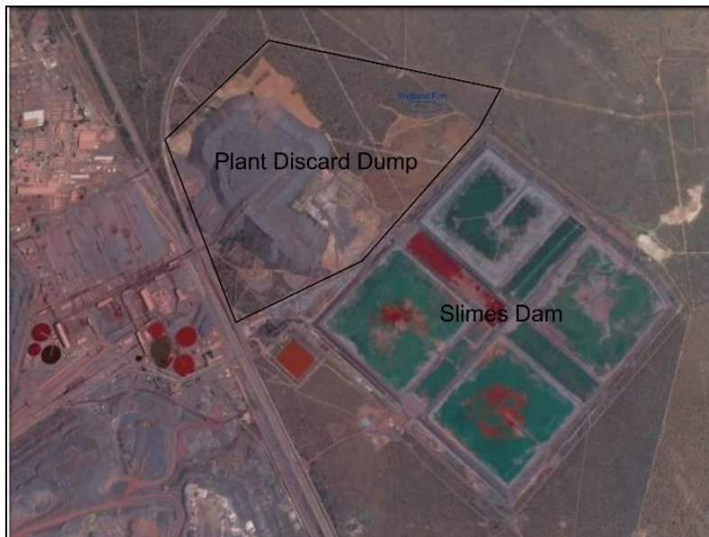
FIGURE 8-10: EXISTING AUTHORISED PLANT DISCARD DUMP AND SLIMES DAM
