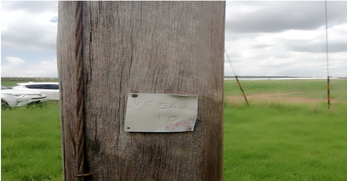
Figure 1: Showing the T-Off line
